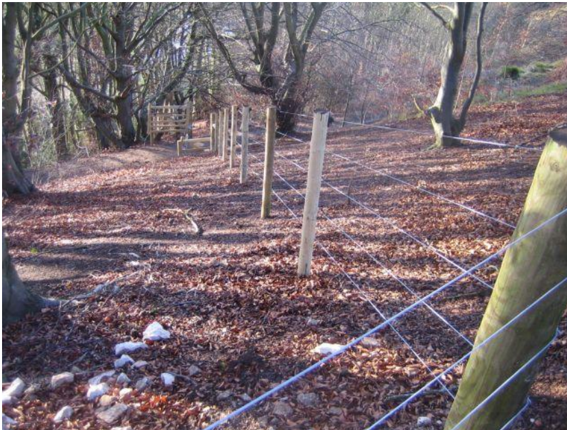
Photographs of the fence
