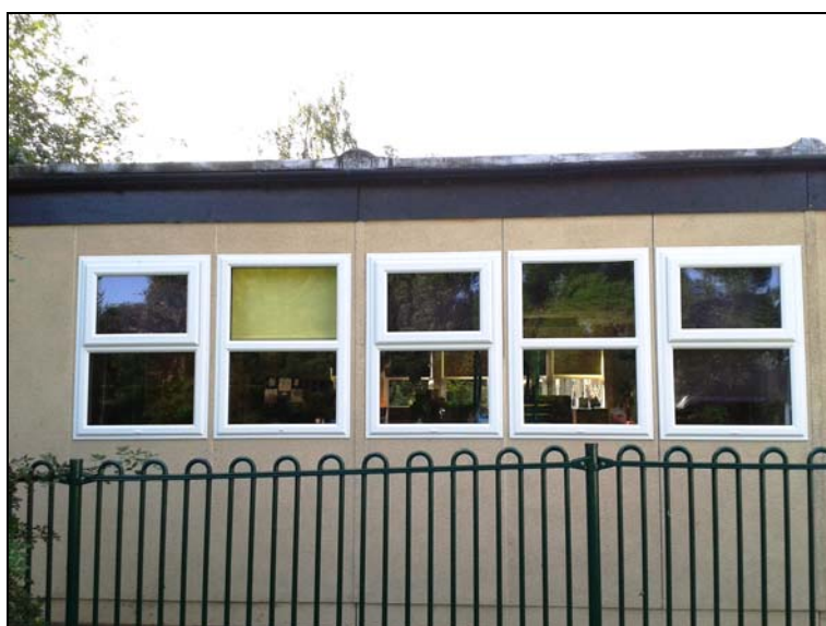
Kempsford Pre-School: Grant towards cost of replacement windows
