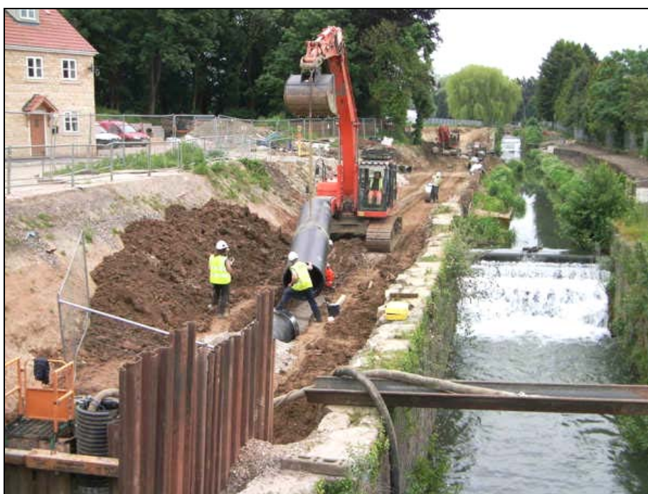
Cotswold Canals Trust: Installation work at Dudbridge, April 2013
