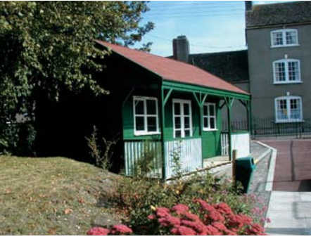
(Top, left) Restored Edwardian tennis pavilion, Wotton-Under-Edge. (See page 17).
